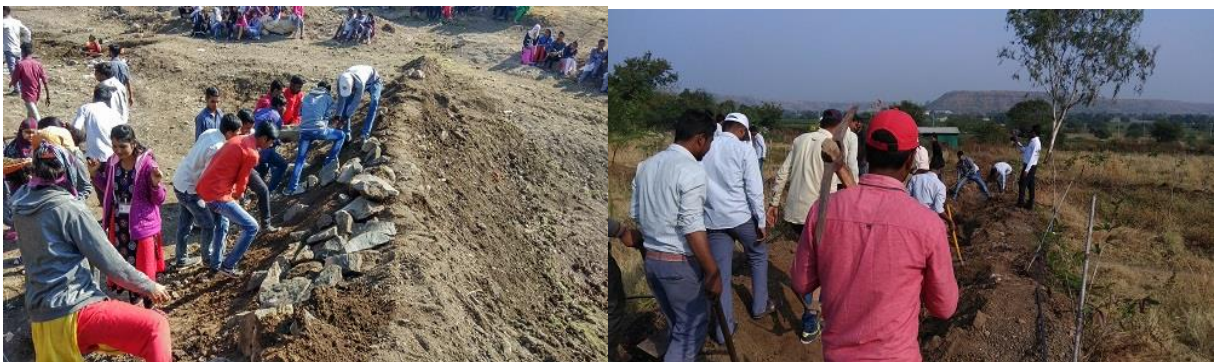
Photo No. 23 Construction of Contour Trenching and Making of Earthen Bunds
